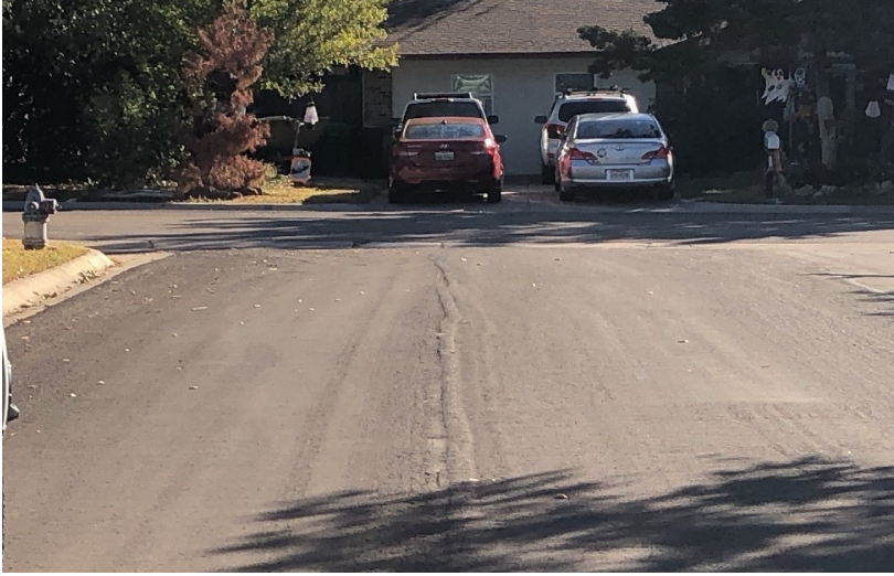
Inconsistent Pavement Joints
